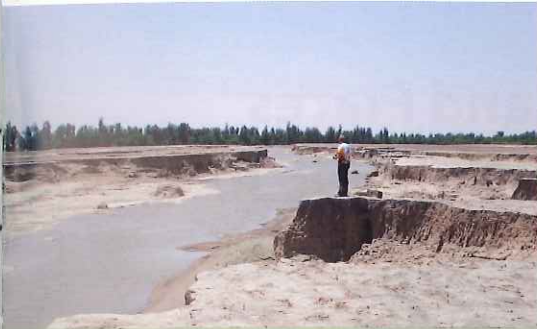
Erosion of gullies in the Birds Point-New Madrid Floodway by floodwaters.
